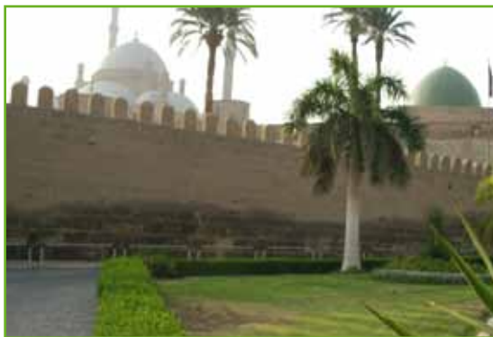
Example for rising damp
