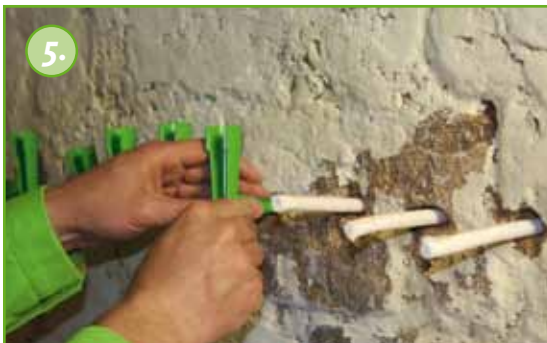
5. The KÖSTER Suction Angles are installed so that the KÖSTER Capillary Rods reach into the supply chamber of the KÖSTER Suction Angles.
