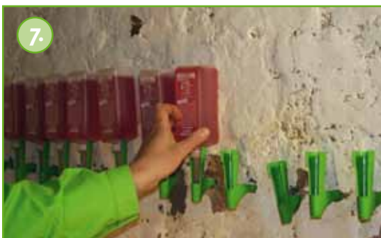
7. The KÖSTER Crisin® 76 cartridges are installed.
