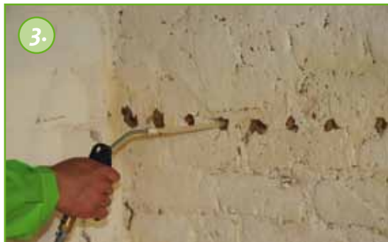
3. The boreholes are cleaned from dust by blowing the dust out of the borehole with pressurised air.
