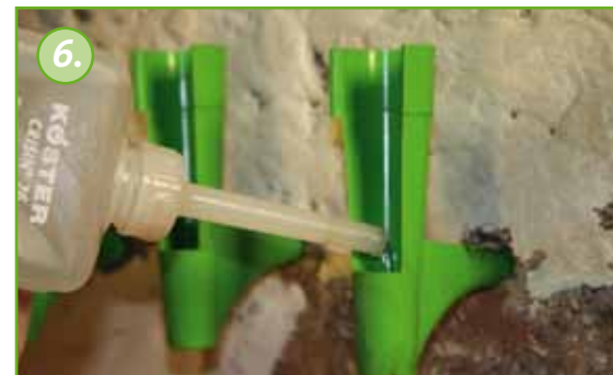
6. The supply chambers of the KÖSTER Suction Angles are filled with water in order to pre-water the KÖSTER Capillary Rods.
