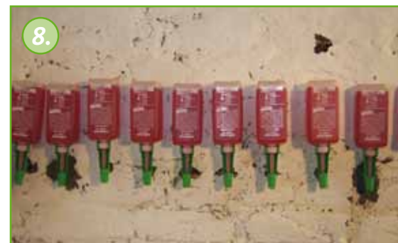
8. The pressureless injection of KÖSTER Crisin® 76 into the masonry starts immediately after the installation of the cartridges.
